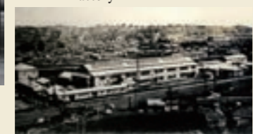
Yokohama factory at the start of operations (Hodogaya-ku, Yokohama)
