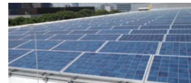
Solar power generation system at the Yokohama Plant
