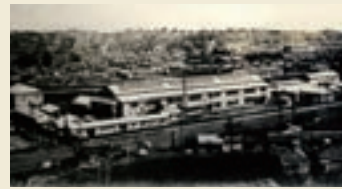
Yokohama factory at the start of operations (Hodogaya-ku, Yokohama)
