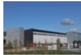
Shiga Ryuo Plant
