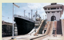
Electric towing locomotive for the Panama Canal
